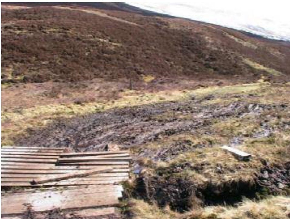
Figure 1 : damaged sections of the existing track
